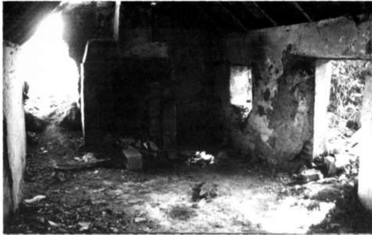
Interior of cottage.
