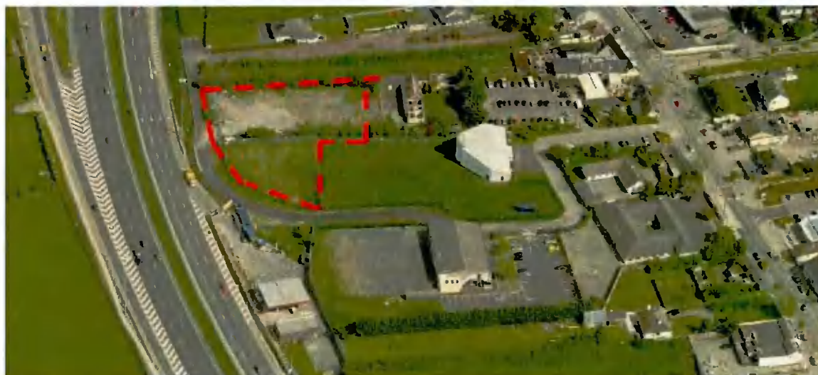
Figure 2-2: Location of prefab units
