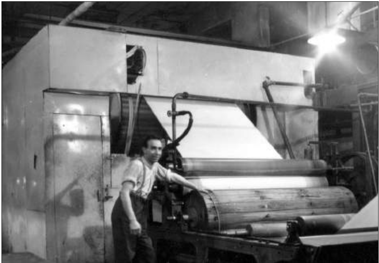
Johnny Timmins, sizer man, is standing at the sizer. The sizer was a vat full of warm size. Paper was put through it and then it was fed under the drying hood where there were drying fans.
