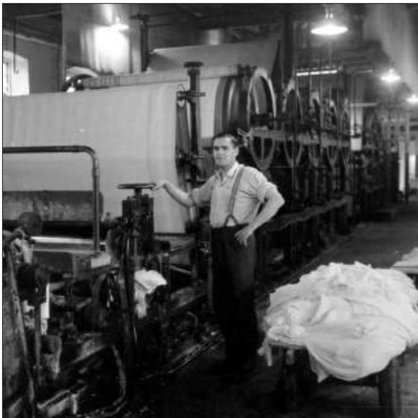
These are the first and second presses. Jim Mullally is standing with his hand on the wheel of the first press. The second press is the felt going up by his head and the paper can be seen going from the second press up onto the drying cylinders. The stuff on the handcart is paper in its wet form. It used be brought back up to the beating loft and reused.
