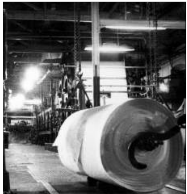
This is the reel machine and a reel, which has just come off number one machine, ready to go onto the calender. To the left-hand side of the pillar are the cylinders of number two machine with the pulp nearer to the left over the drying cylinders.
