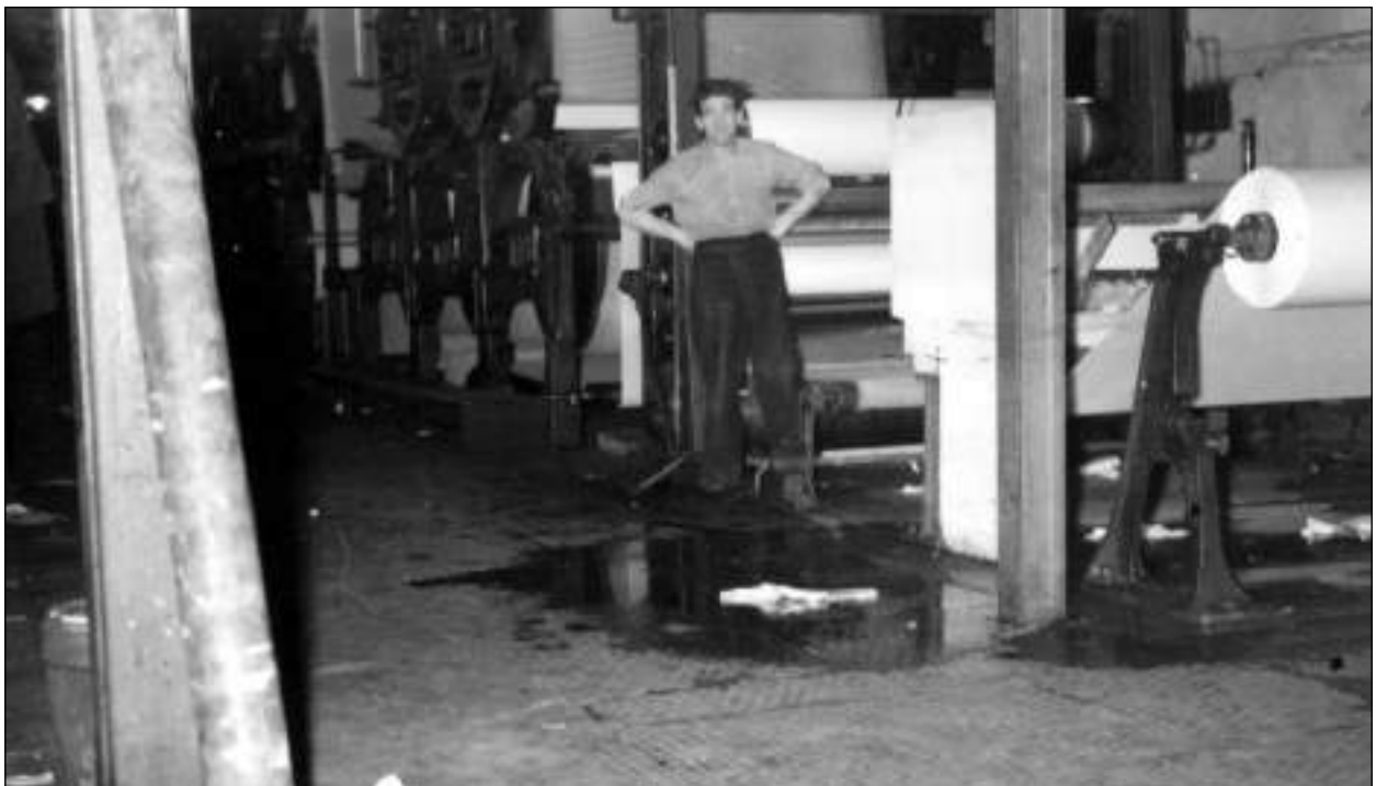
This is a view of the second stack of drying cylinders and the stack of calenders, where John Quinn is standing. These are steel rolls and the paper had to be laced through them and then it came underneath the spray and up onto a reel.
